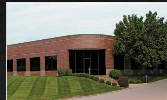
STEEL PREPARATION FACILITY St. Charles, Missouri, USA
