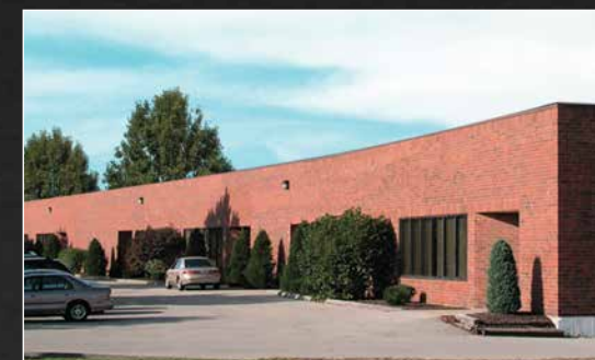
TURRET MANUFACTURING FACILITY Chesterfield, Missouri, USA
